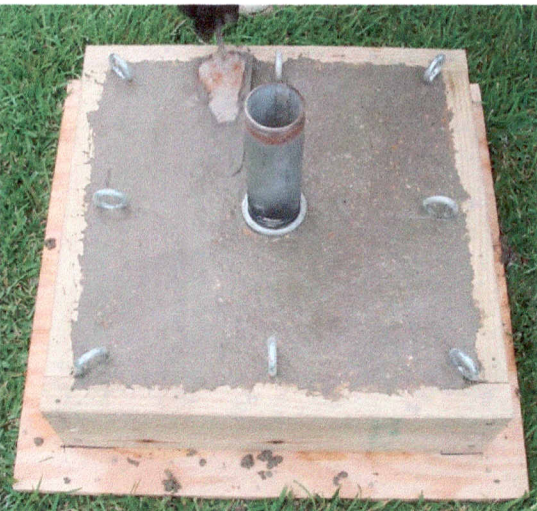
Eight Eyebolts Installed
