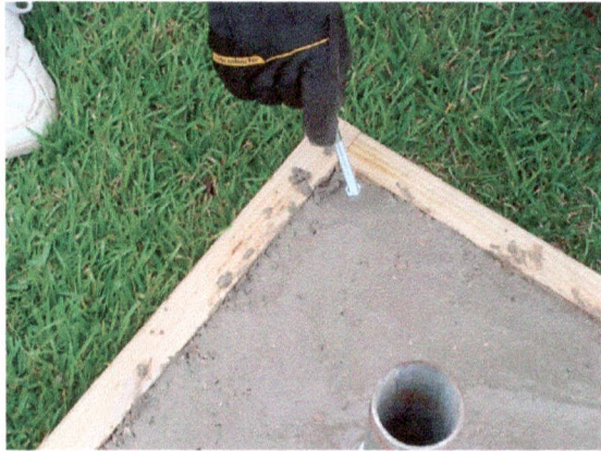
Install Eyebolts at an Angle
